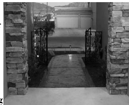
Zero-step threshold at entrance of certified home by Blue Ribbon Builders, El Paso, TX.
